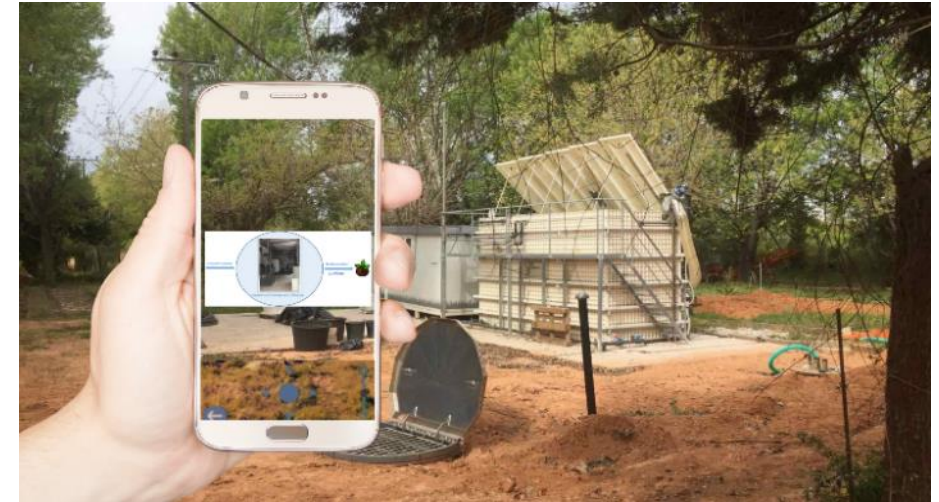
The view from the AR app next to the Athens sewer mining bioreactor
